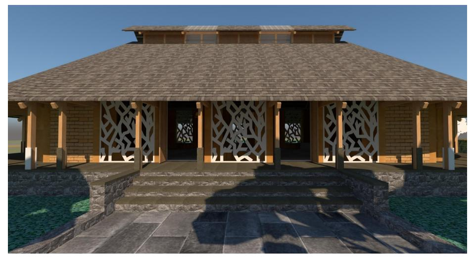
Behind the verandah columns, one sees both mud concrete masonry and monolithic earthen walls. That is broken by jaali screens and doors.
