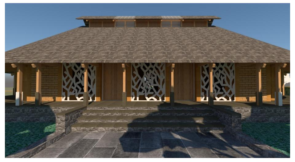
The KC is approached through a front stone paved court. A stone masonry plinth raises the structure a couple of feet above the ground.
