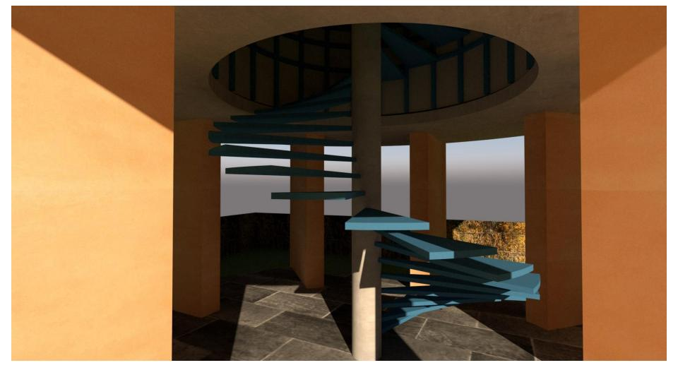
At the centre of the tank base, a spiral staircase rises up to access the top of the tank
